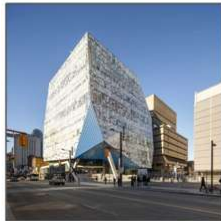
Fritted glass on the facade of Ryerson University student Centre, Toronto, Canada
