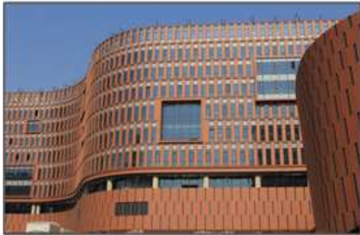
Terracotta tiles on the facade of Bund House office complex, Shanghai, China
