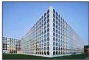
FRP panels on the facade of Ravel Residence, Student housing
