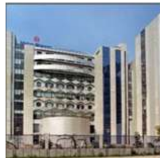
Composite Aluminium Panels on DMRC Metro Bhawan, New Delhi, India
