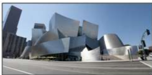
Stainless Steel cladding on the facade of Walt Disney Concert Hall, Los Angeles, USA
