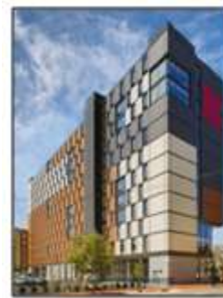
Rain-screen cladding façade in Rutgers University Camden Graduate Student Housing, USA
